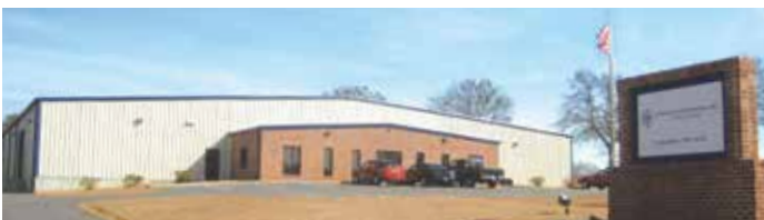
AIRCRAFT COMPONENTS AND GSE MRO FACILITY
